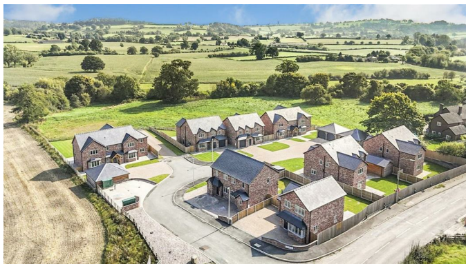
Aerial Additional Photograph
