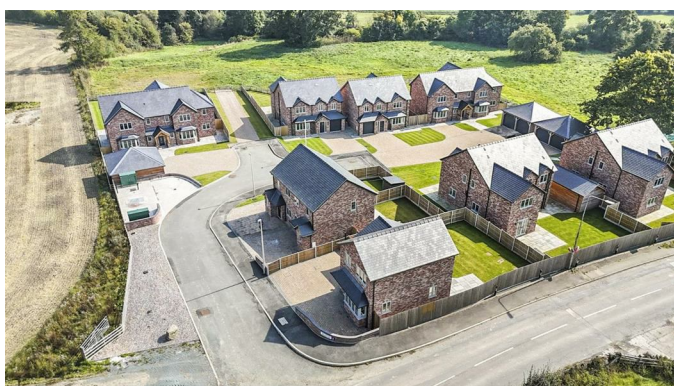
Aerial Photograph Of Development
